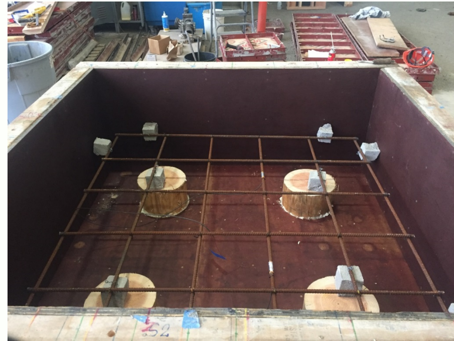
Typical Timber Pile Footing
